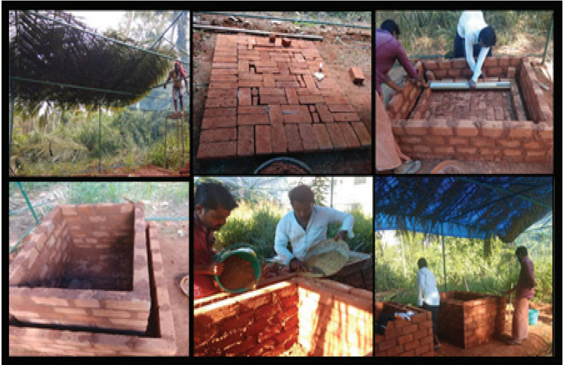
Plate 1. Construction of ZECC
